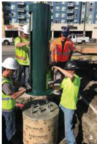
Step 2: Install base section cabinet of the CityPole™ onto the foundation and secure.
