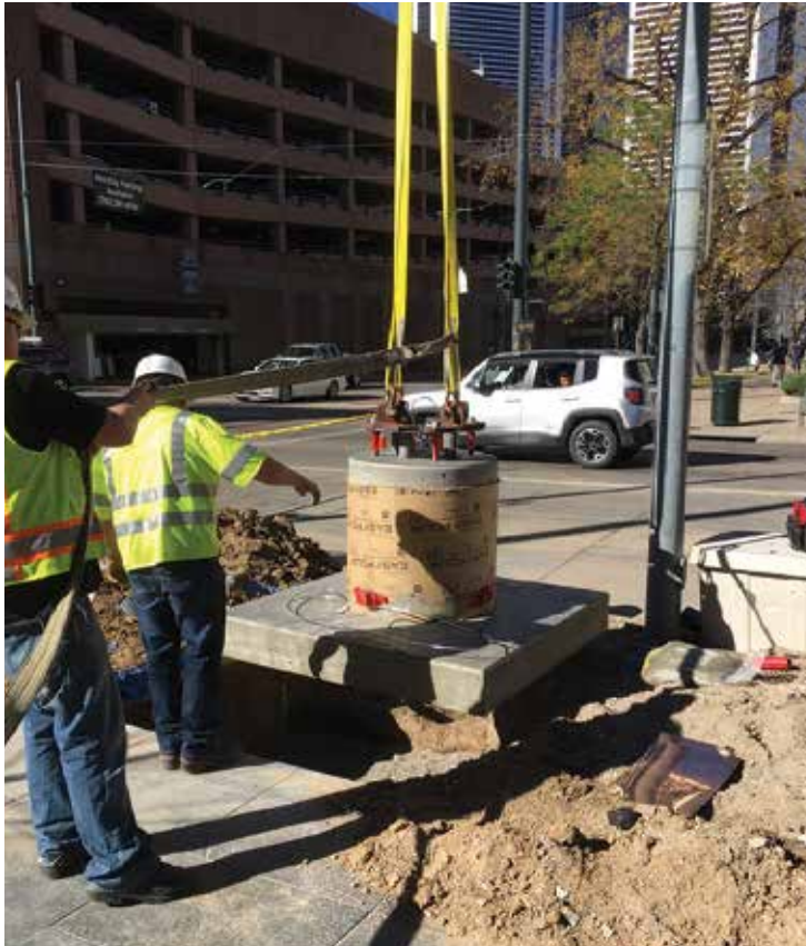
CityPole® foundation systems can be engineered for existing and future loadings and fast installation.
