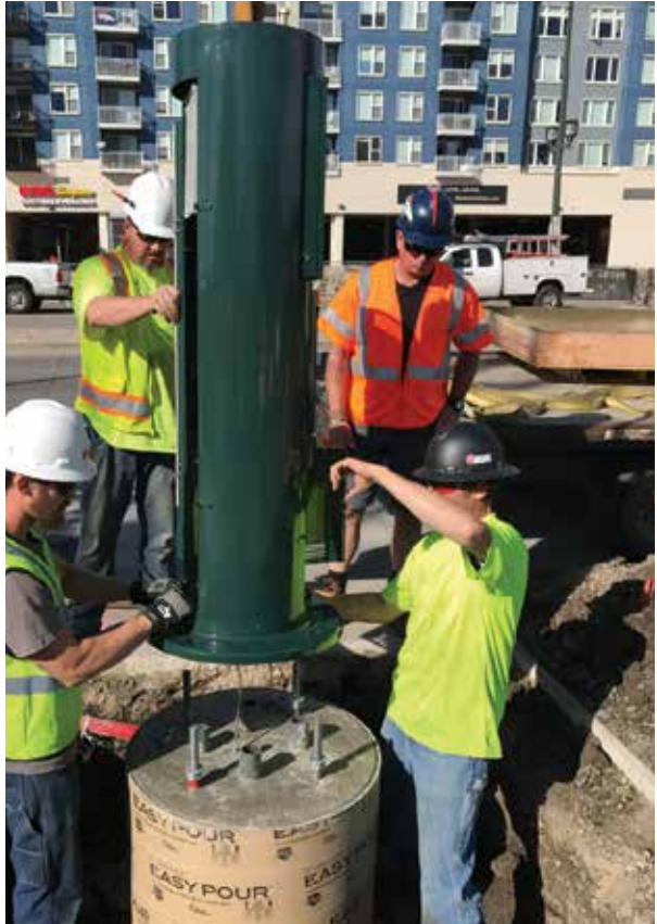
CityPole® foundation systems can be engineered for existing and future loadings and fast installation.
