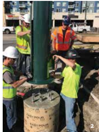
Step 2: Install base section cabinet of the CityPole® onto the foundation and secure.
