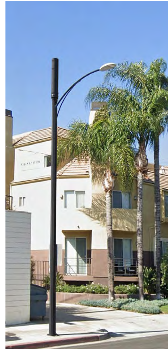
5G Top Mount Shroud on Octagonal Support Pole
