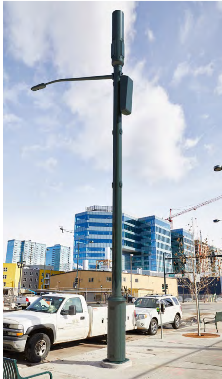
Mid-Power Backpack on Round Support Pole with Base Cabinet
