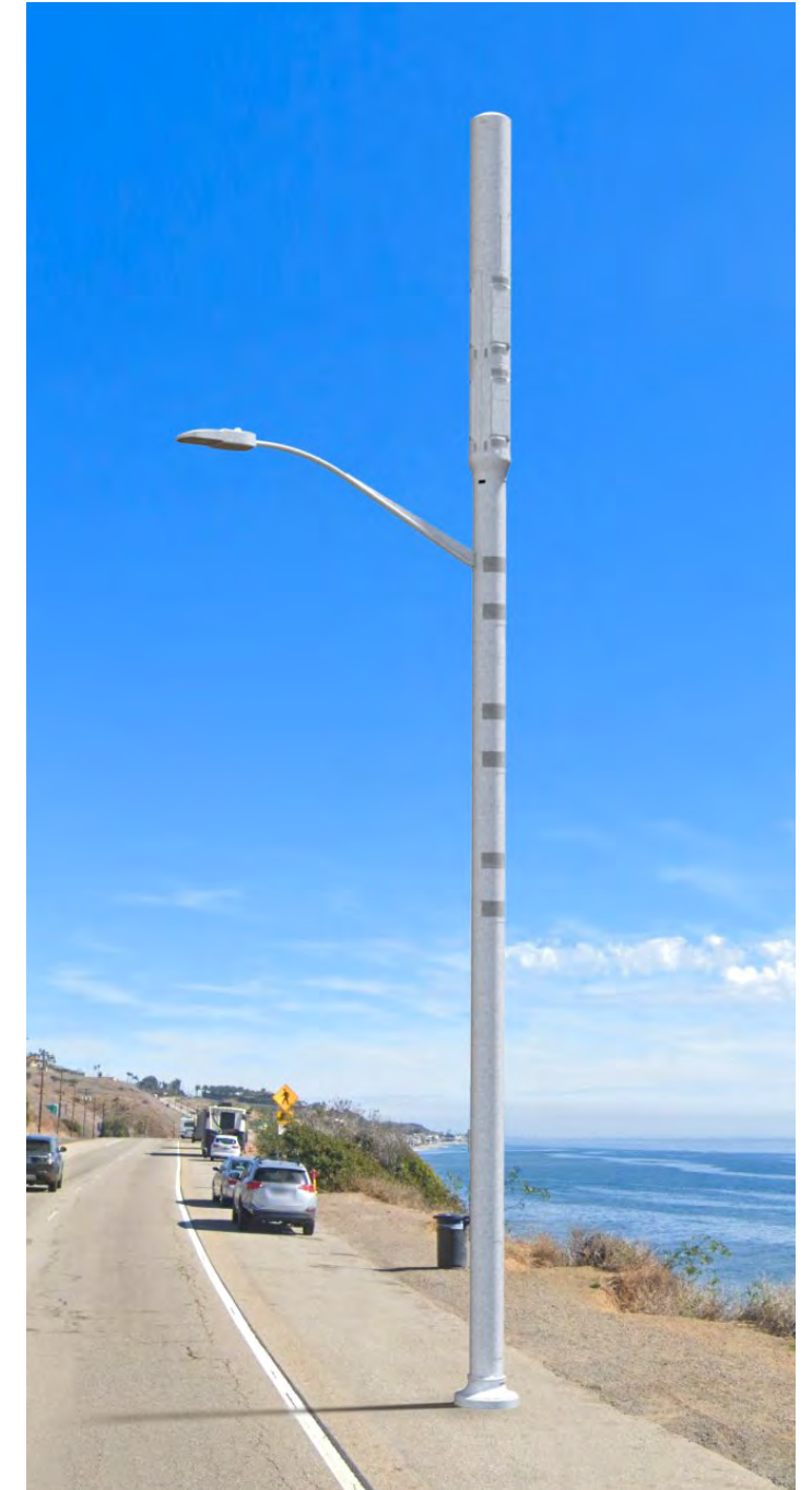
Ø12.75" Multi-Tenant Pole with Faux-Tapered Cobra Light Arm
