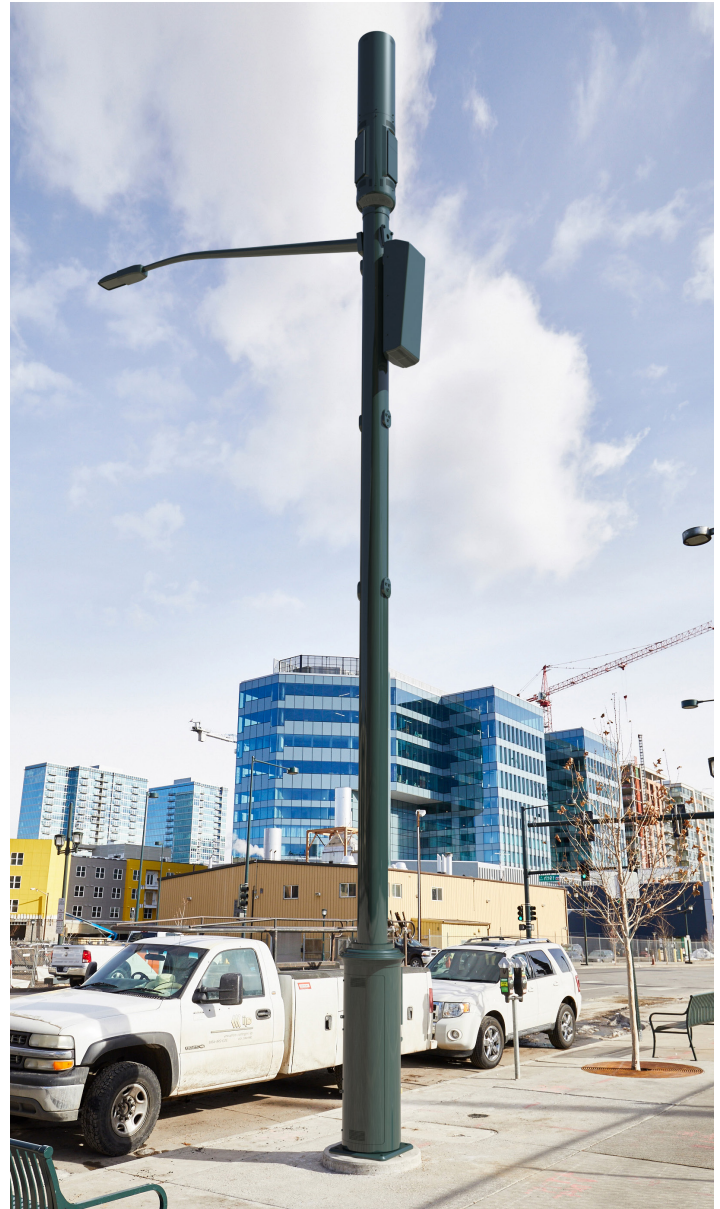
Mid-Power Backpack on Round Support Pole with Base Cabinet
