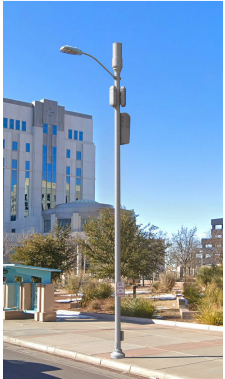
High-Power Backpack on Round Support Pole
