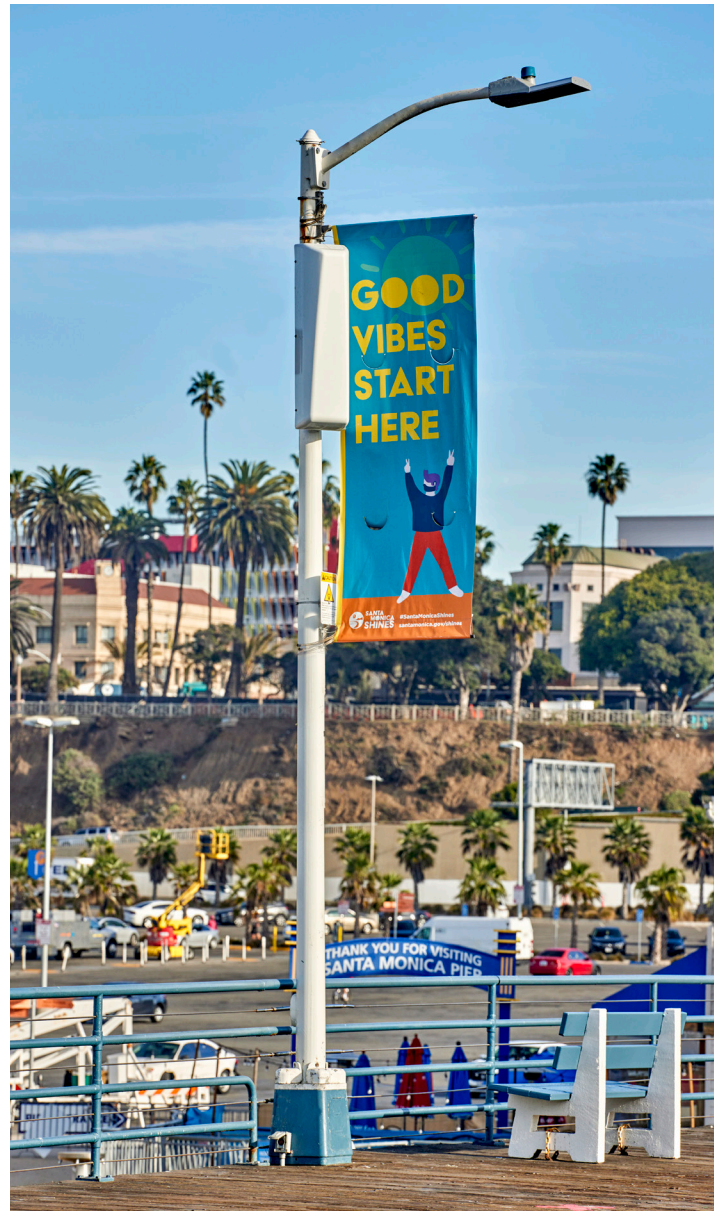
Low-Power Backpack on Existing Round Pole
