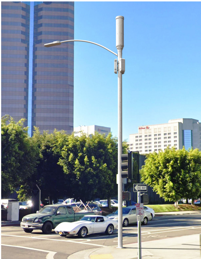
Low Profile Modular Side Mount Shrouds on Round Support Pole
