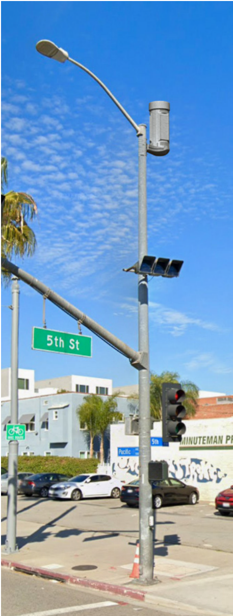
Traffic Pole Side Arm Mount
